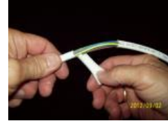
Open two "windows" in sheath
