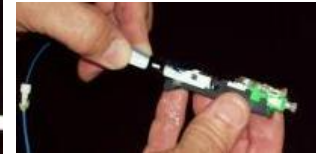
Add connector ( SOC, Splice )
